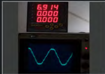
Supply current wave form showing harmonics supported by harmonics meter above
